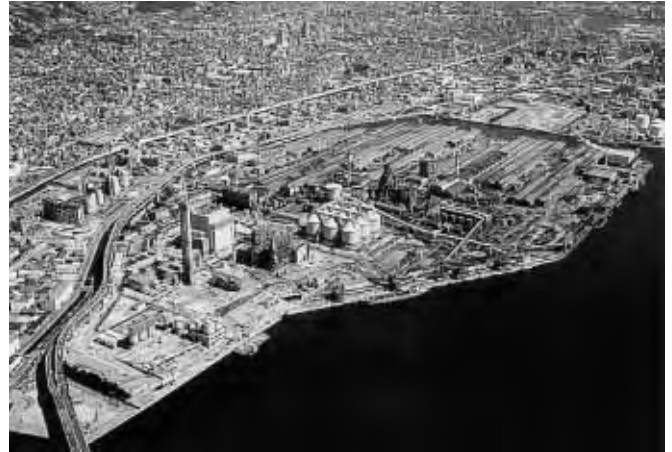
Photo 1 View of Kobe Steel's Shinko Kobe Power Station
